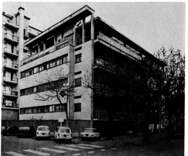
37. Giuliani Frigerio Apartment Block, corner view from which a planar reading is revealed.
